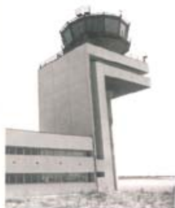
1 CONTROL TOWER Architect: Manfredi Nicoletti Completed: 1977 Address: Catania Airport
